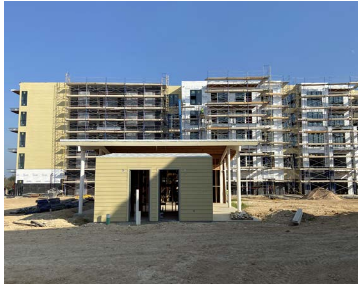
Scaffolding for stucco install
