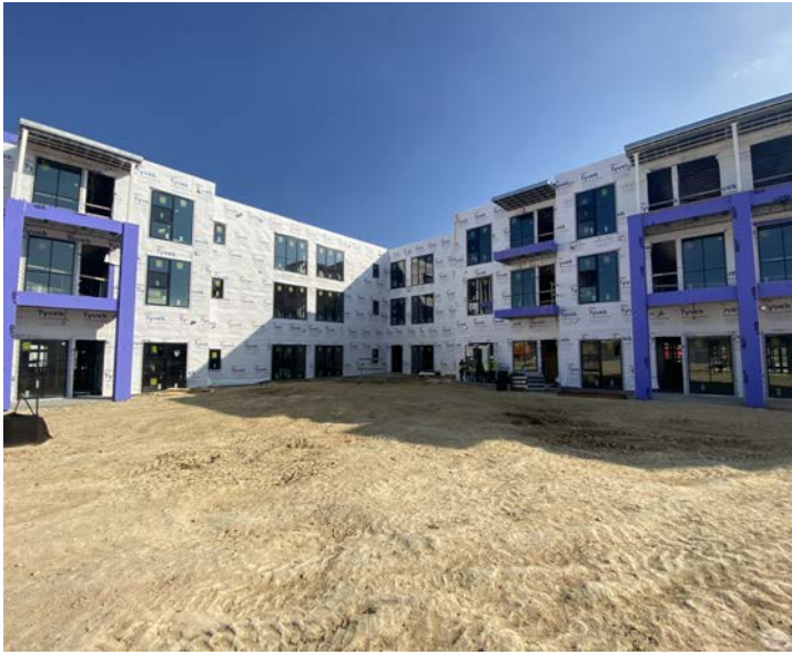
AL ready to receive exterior finishes
