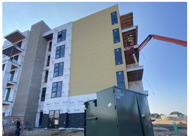
Siding installing on IL
