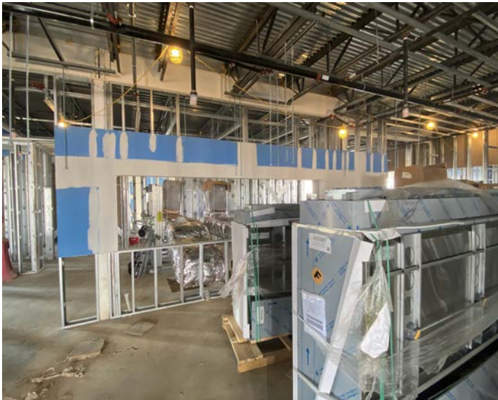
HVAC duct & equip ready for install
